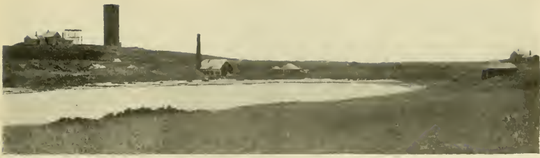
Standpipe—Wannacomet Water Works
